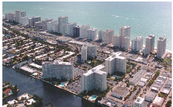
Galt Mile Condominium Association, a 27 building, 6,400 unit association that would be required to retrofit with sprinklers.
